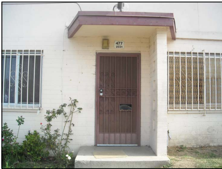
Typical security lighting found at dwelling unit entrances within Jordan Downs public housing complex.
