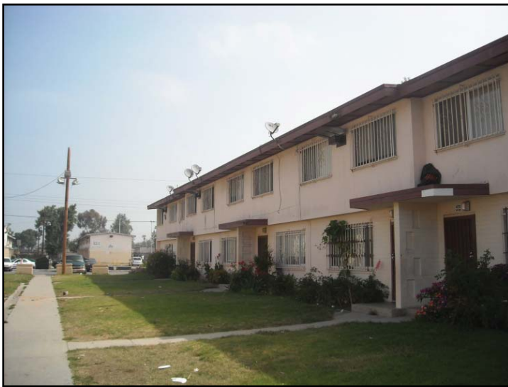
Typical security lighting found on the front and rear entrance sides of residential buildings within the Jordan Downs public housing complex.
